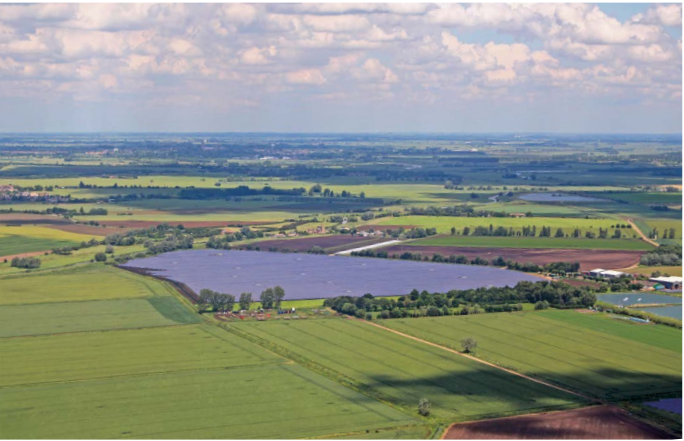
STOWBRIDGE, GROSSBRITANNIEN 24,3 MWp
