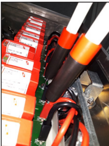
Example: VAT between CH3(+) and PE
